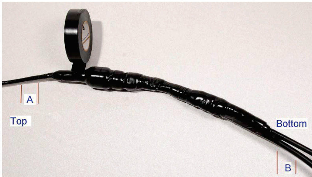
Figure 105 Wrapping PVC tape around the GPS adapter cable joint
